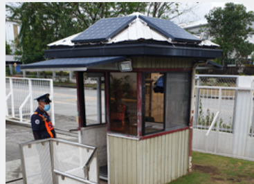
Installation of Solar Panels at the Security Post
